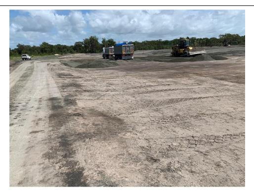
Photograph 3 – Placement of first layer of imported material on site (Lot 109) on 17 February 2020.
