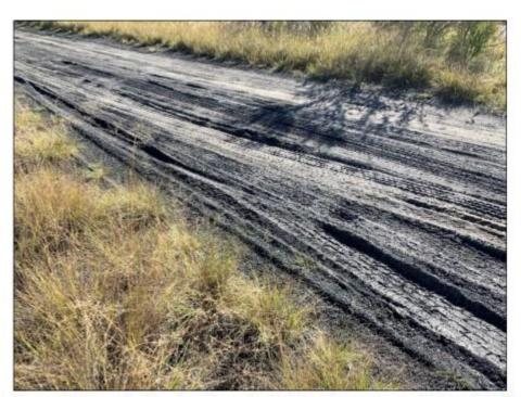
Figure 13: Unsealed track with coal reject / carbonaceous siltstone (2019)
